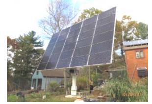
Solar Tracker – with Bifacial Panels & Other Special Features
